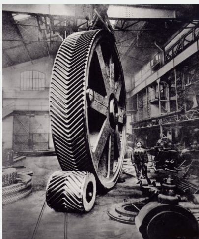
Set of gears with inverted V shape teeth Copyrights : Citroën Communication
